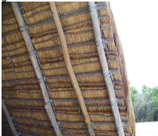
Classic example off tight thatching on a hut I photographed in Hawaii
